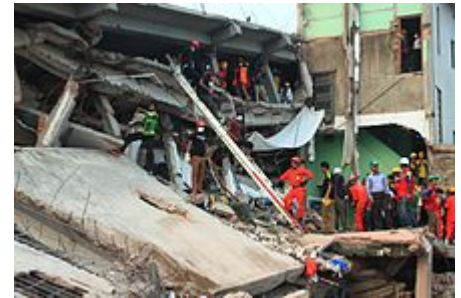
Side view of the collapsed building
